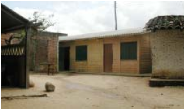
Original home with unfinished construction
